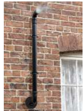
Installed to prevent nuisance plumbing across the window
